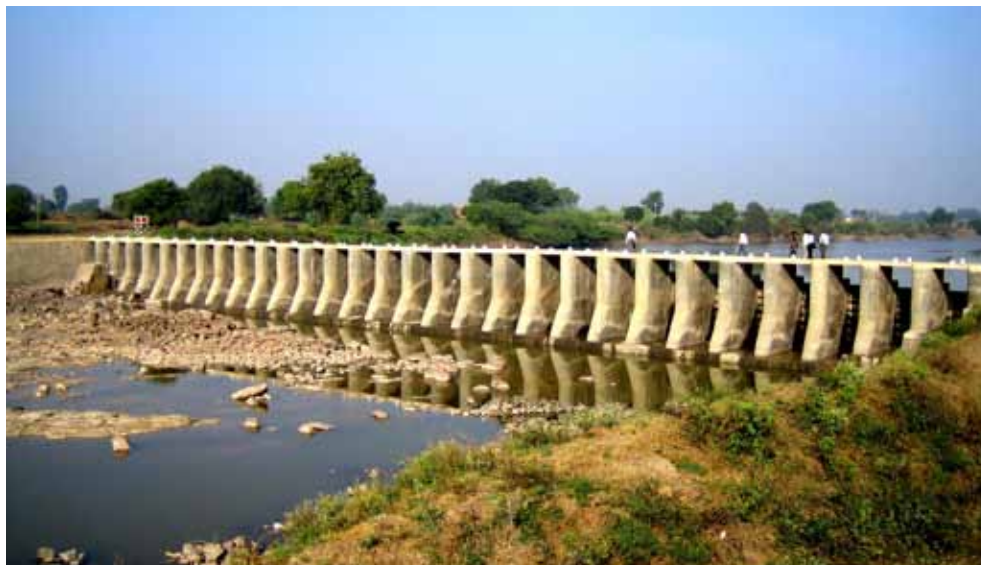
Figure 1: Downstream side of Bolegaon KTW (Photo credit: Olaf Verheijen)
