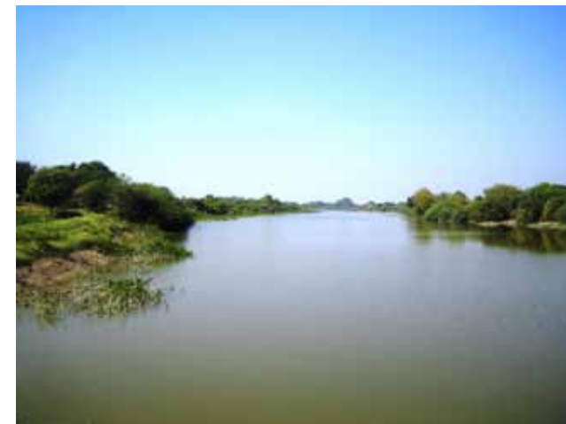
Figure 2 and 3: Piers with installed shutters and bridge (upper) Reservoir area upstream of KTW (below) (Photo credit: Olaf Verheijen)
