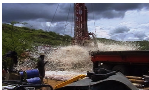
Figure 24. Drilling of deep boreholes, to increase access to a larger volume of stored groundwater reserves.
