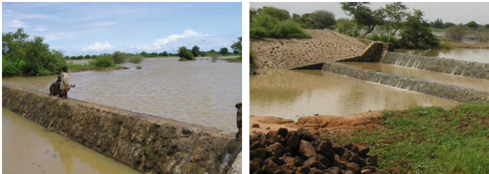
Figure 35. a) Water in water-spreading weir; b) Water-spreading weir in Kalfou (Tahoua region, Niger) (Photos: GIZ/Aboubacar Mounkaila).
