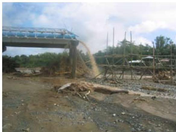
**Flood-damaged main pipe for potable water for the City of Iloilo.**
