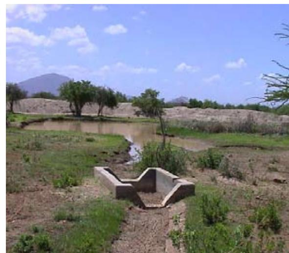
*Photo (left): Silt trap intercepts sediments from the rainwater*
