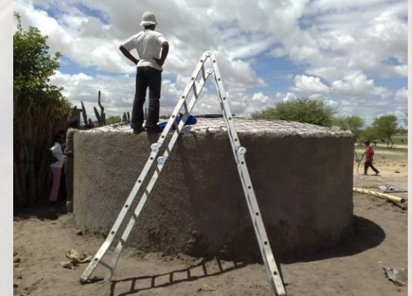
roof catchment with ferrocement tank
