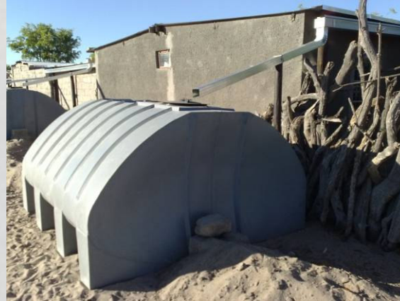
roof catchment with plastic tank
