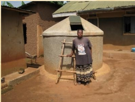
Subsidized 4000-liter ferrocement tank
