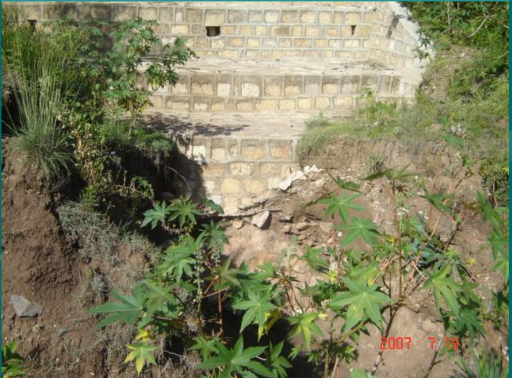
Gully created as a result of the culvert – in Dhangego KA of Kersa
