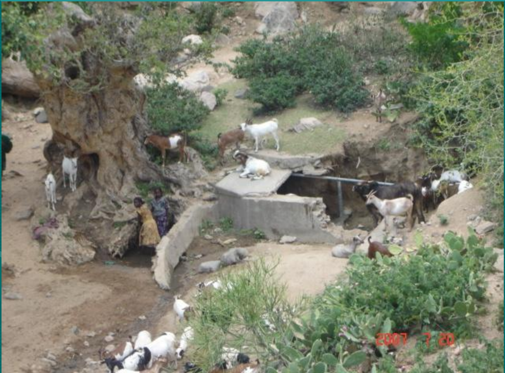
Developed spring collection chamber and takeoff is destroyed by flood – Lege Biyo in G. Oda
