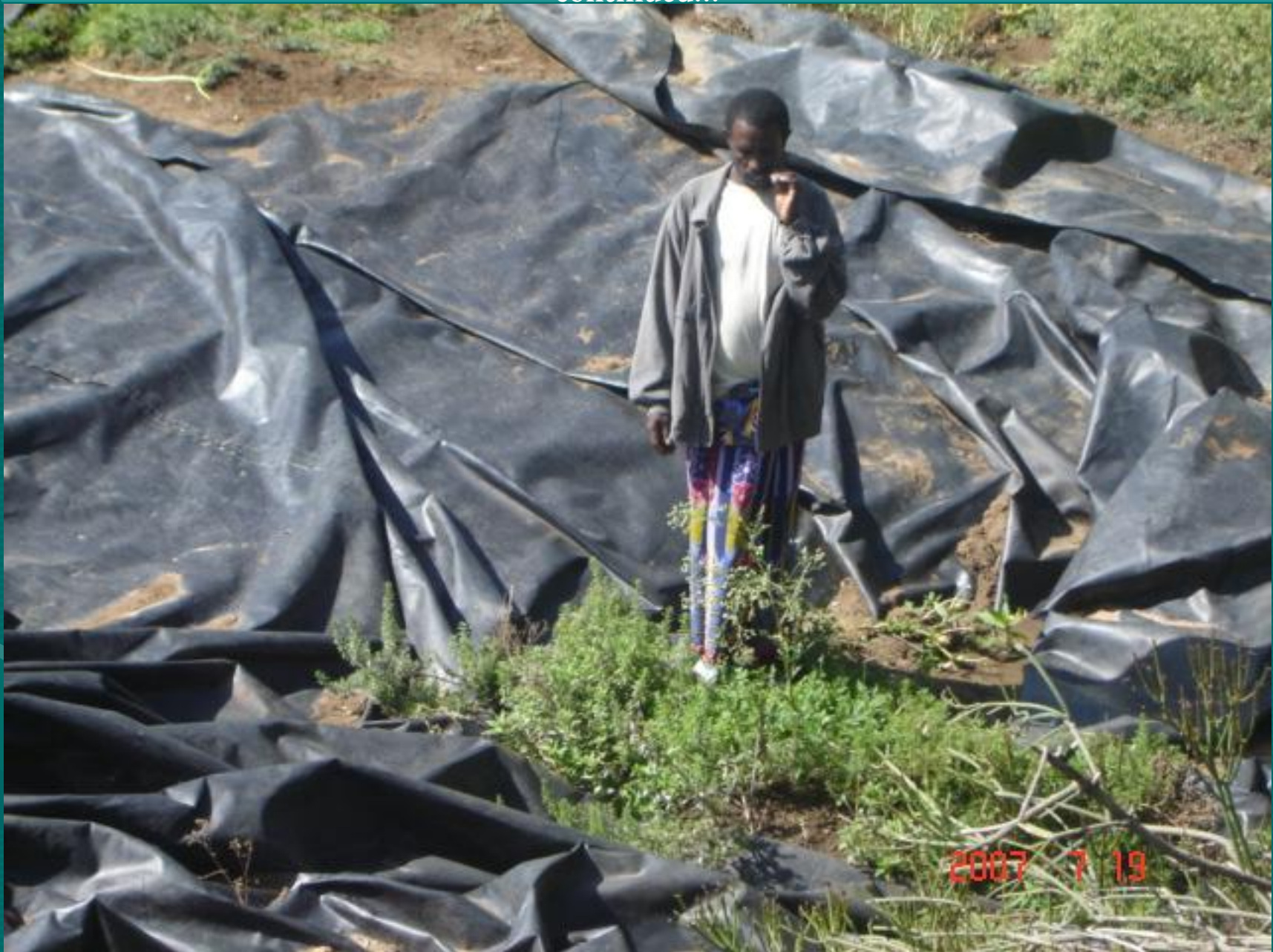
Not properly constructed HH WH (pond) with geo-membrane lining G. Goro Seka continued...
