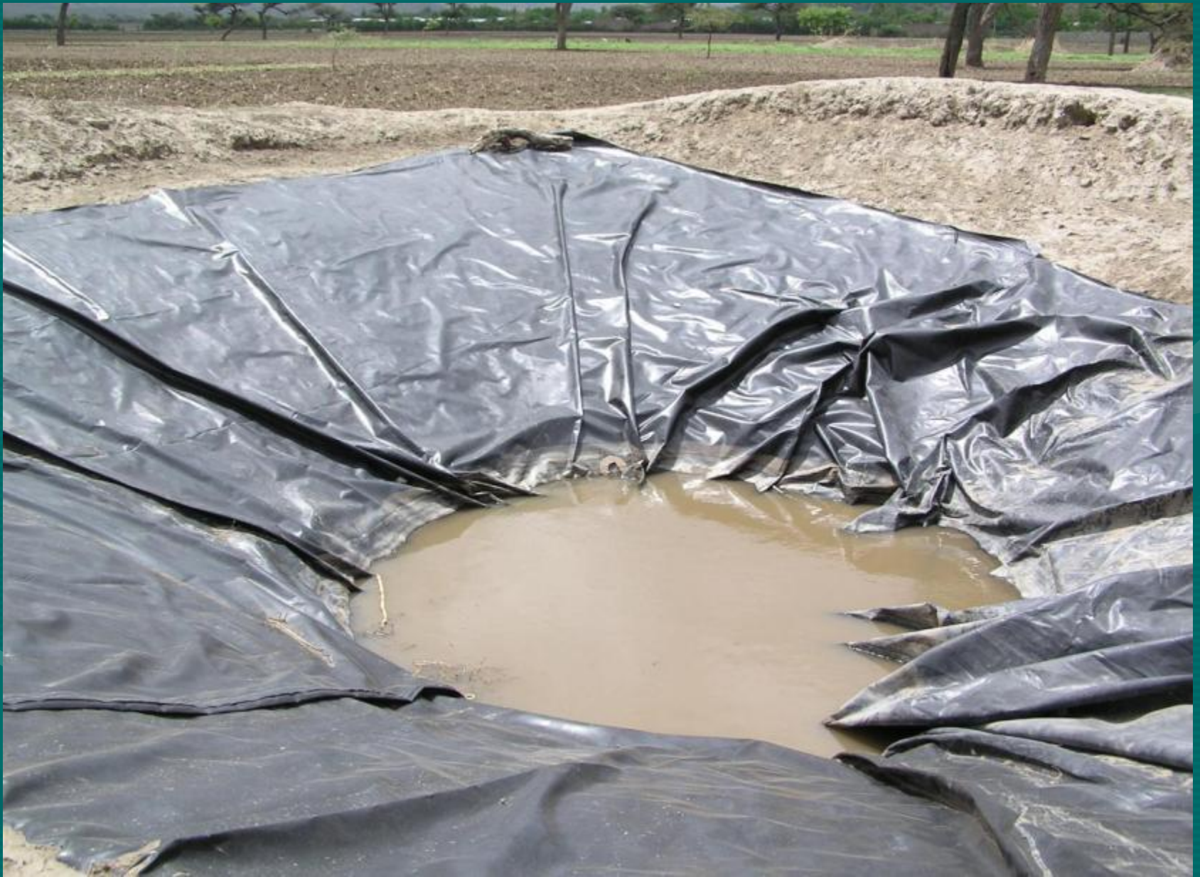
Poor plastic lining
