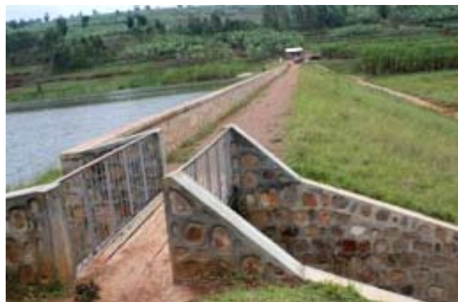
Figure 11 Waterways drain water to the valley dam reservoirs. It is used in dry seasons for hillside irrigation of crops, Rwanda.
