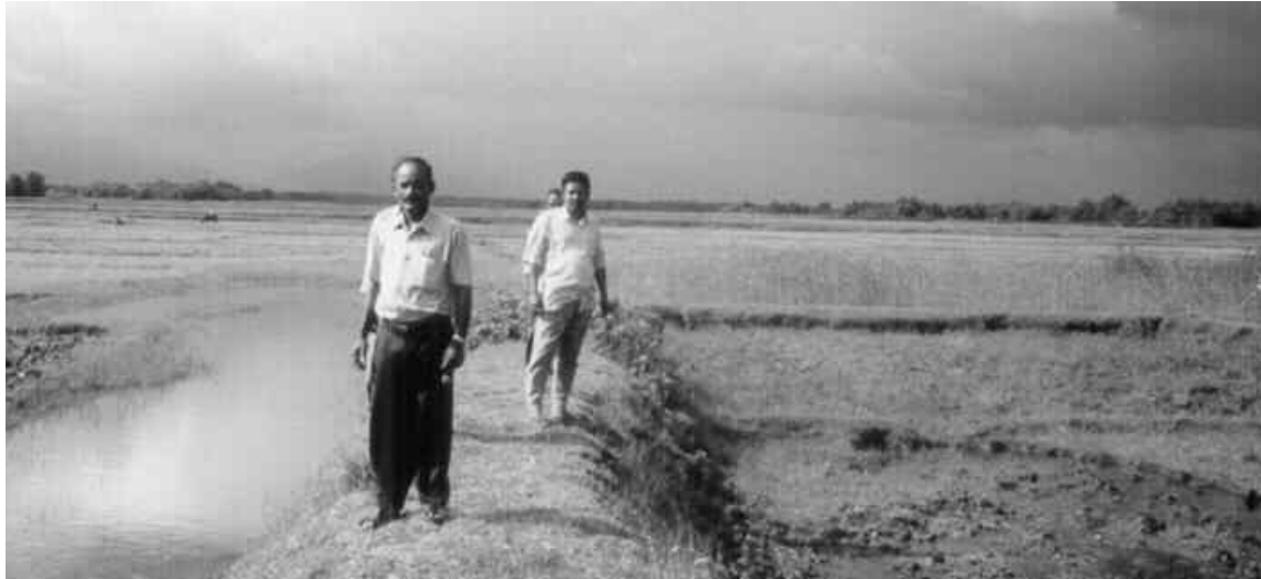
Earthen gully plug – diverting water and raising groundwater tables
