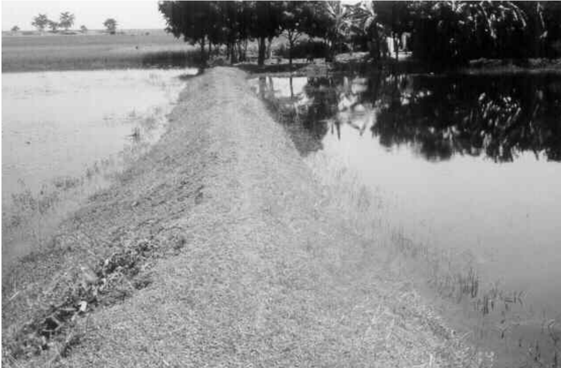
Ponds created by putting a cross bund in borrow pit
