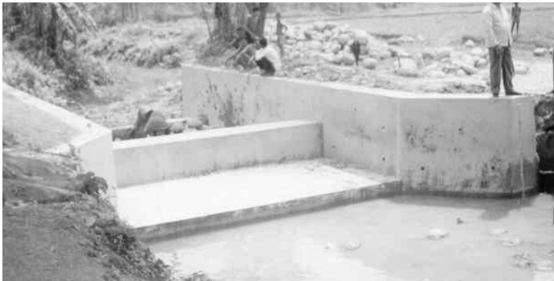
Plastered masonry gully plug – raising groundwater levels
