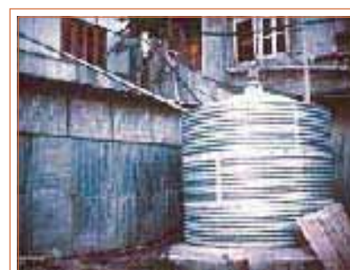
A storage tank made of galvanized iron sheets
