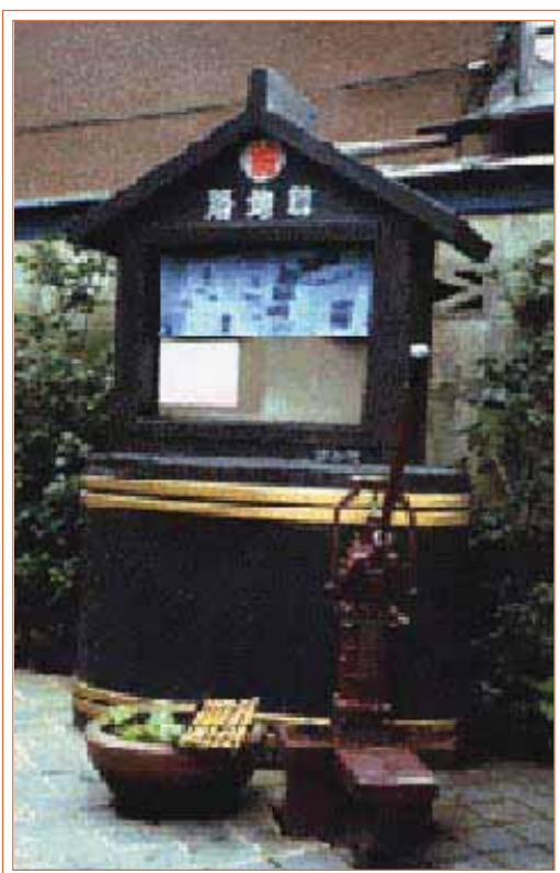
'Rajison' a simple and unique rainwater utilisation facility at the community level in Tokyo, Japan.
