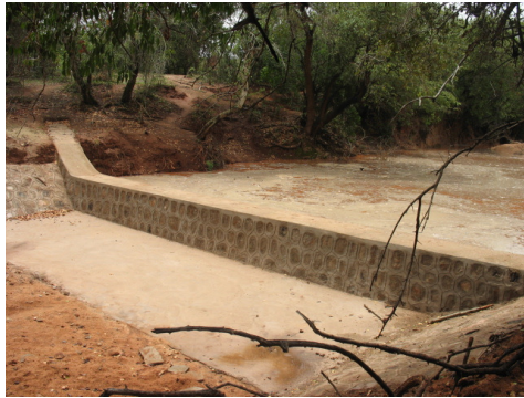
Photo 7: Sand dam site after first flood event in Borana, Ethiopia (ERHA, 2008).
