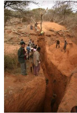
Photo 3: People excavating a trench (RAIN, 2007).
