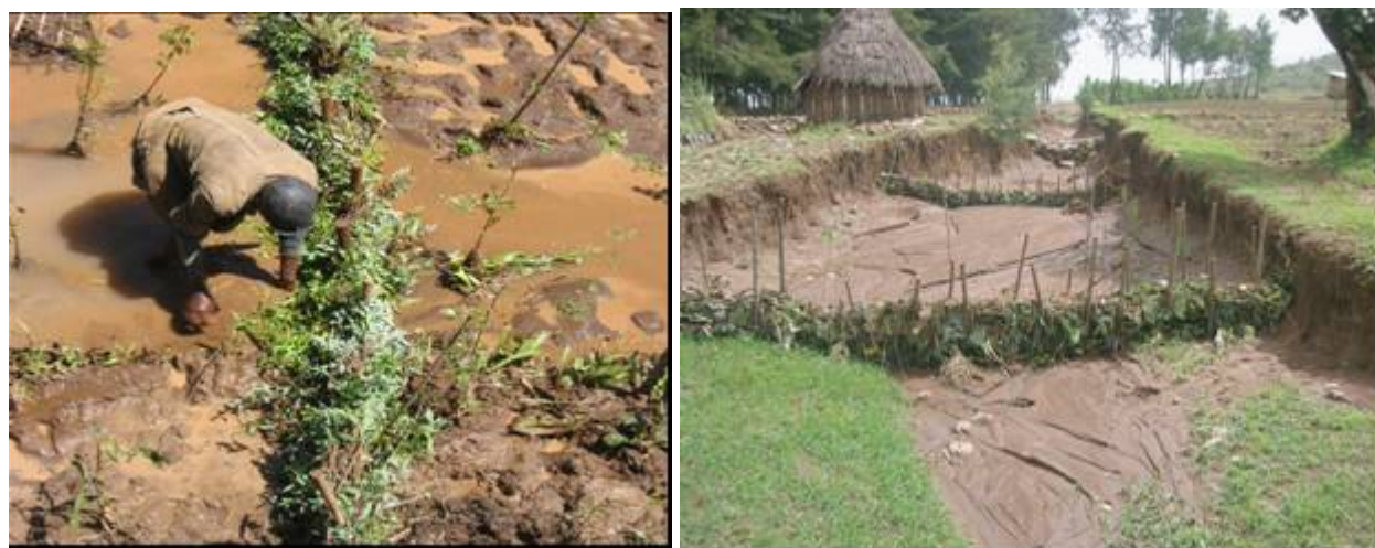
Plate 10. Bundles put across the gully bed and supported with poplar and willow stems
