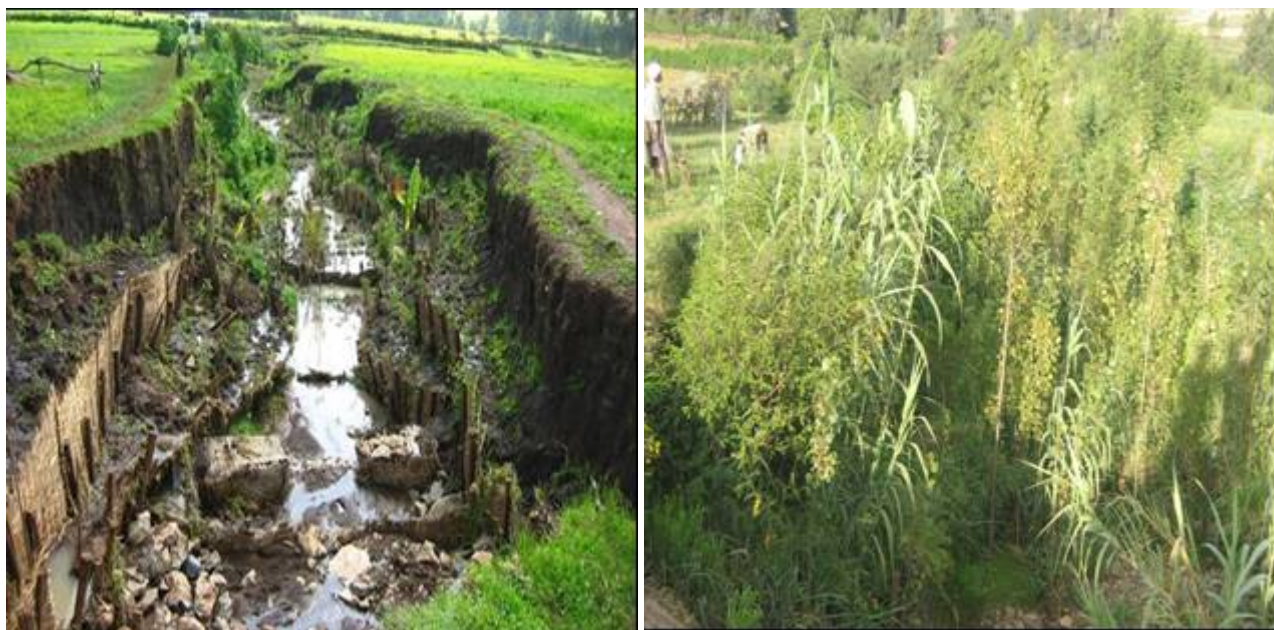
Plate 13. Protecting gully sidewall using bamboo-mat retaining wall.
