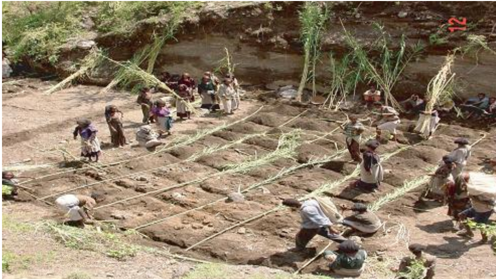
Plate 11. Planting of elephant grass by layering to rehabilitate gully bed
