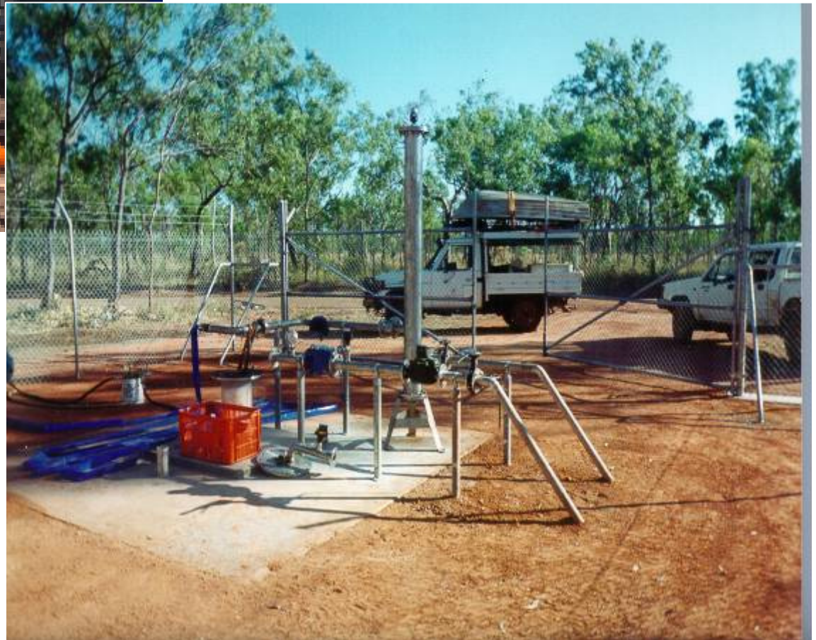
Groundwater ASR for drinking water supplies at Warruwi, NT
