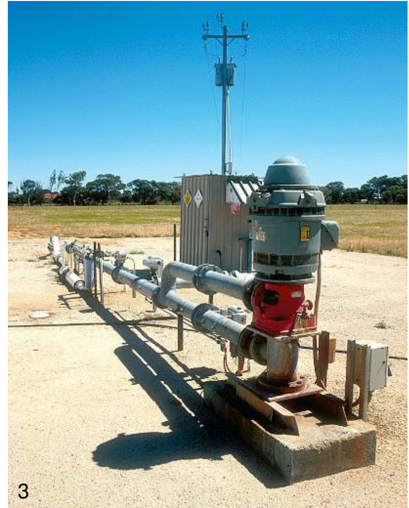
ASR Injection well
