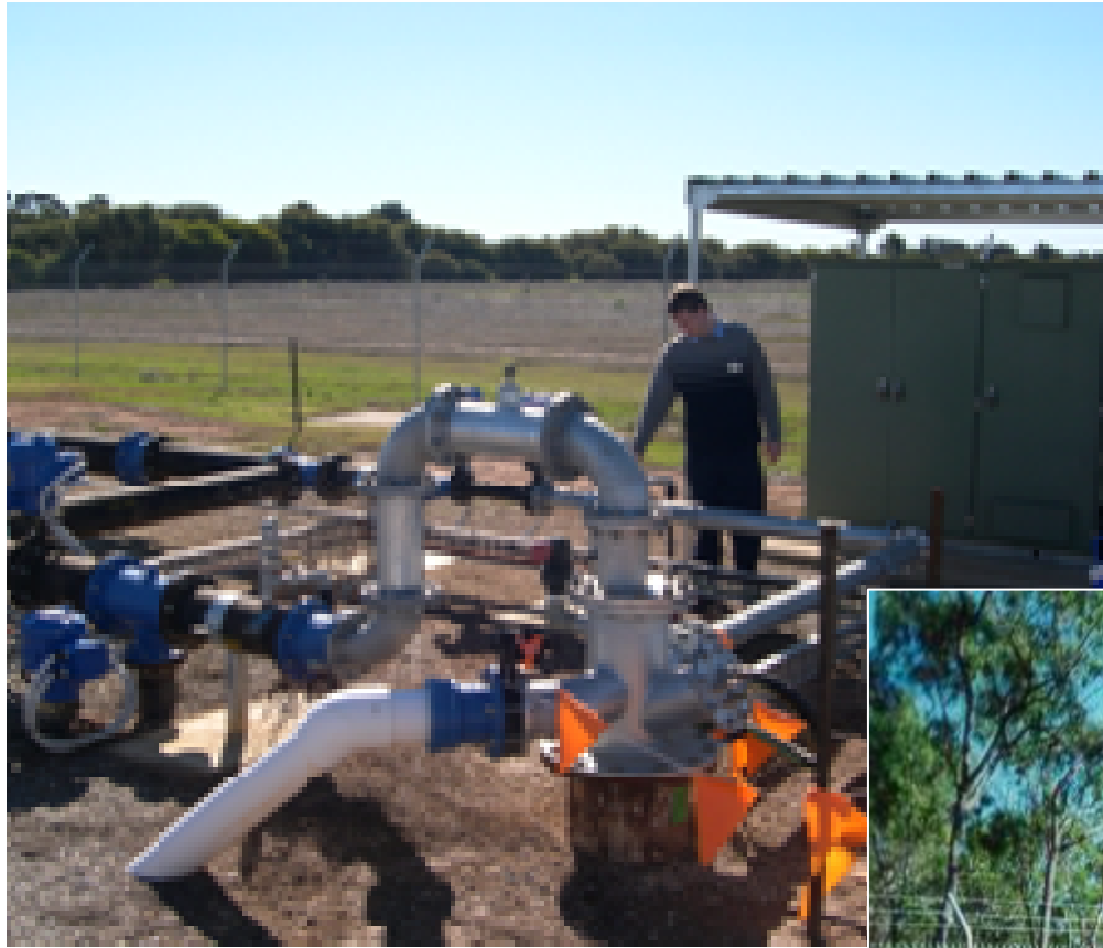
Stormwater ASR for industrial water supplies (Salisbury, SA)
