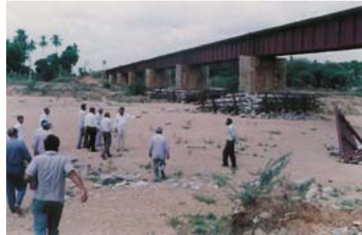
Figure 3: Railway bridge foundation frequently being repaired due to sand mining across Uttara Pinakini river in Gauribidanur taluk, Karnataka, 2002. (Hemalatha, A.C. et al. 2005)
