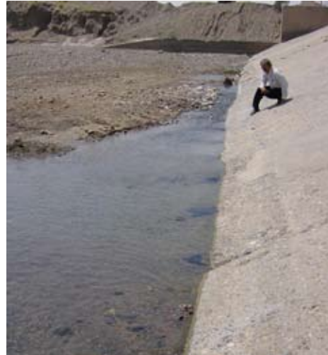
Figure 3: Water emerging from weepholes
