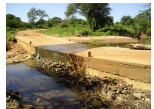
Figure 3: Irish bridge (Source: Nissen-Petersen, E, 2006)
