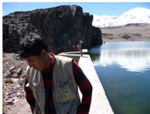
Figure 1: A retention dam at Lago Palcacocha, near the Coropuna Glacier
