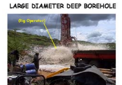
Figure 4: Drilling of large diameter deep borehole
