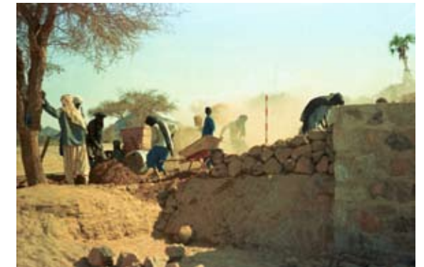
Figure 2: Construction of diversion works
