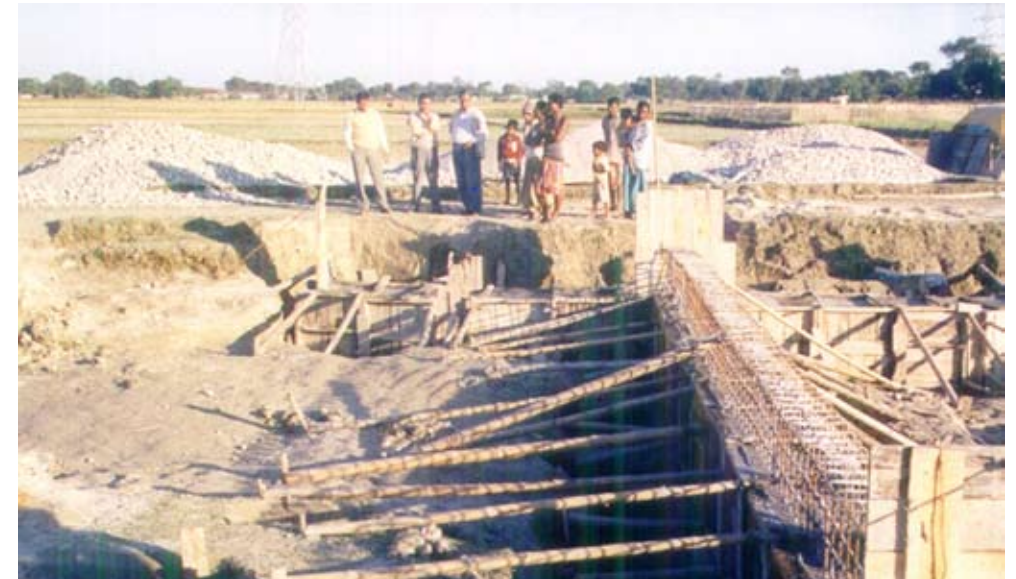
Figure 2: Constructing a gully plug to retain groundwater
