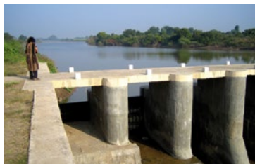
Piers with installed shutters and bridge (upper) Reservoir area upstream of KTW (below) (Photo credit: Olaf Verheijen)
