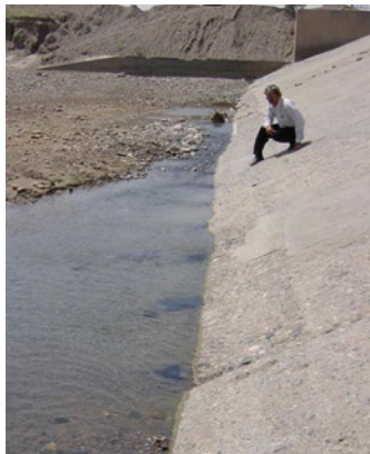
Water emerging from weepholes
