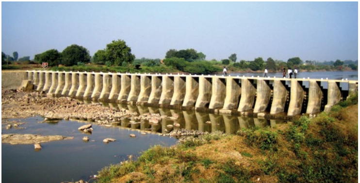
Downstream side of Bolegaon KTW
